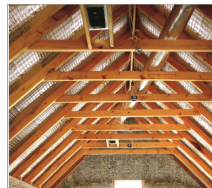
Example installation in a new construction application where the radiant barrier is pre-laminated to the roof decking
